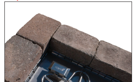
Install the insert
